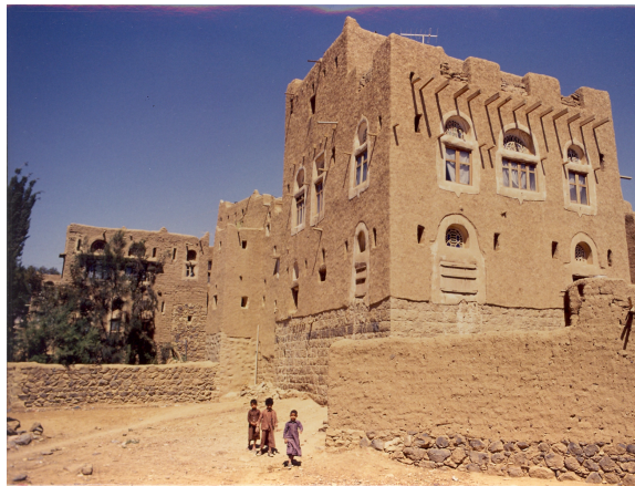
Figure 2: Private house built in the town of Amran in Yemen in 1985 Photo: CRATeere/EAG
